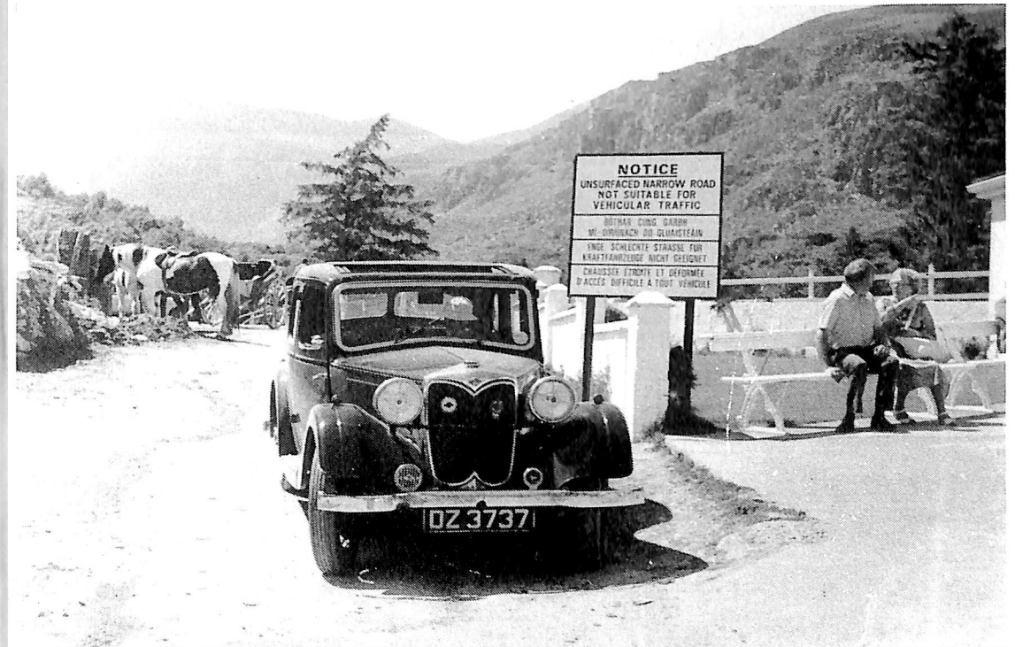
A road which is unsuitable for vehicular traffic really should have a sign at each end!
